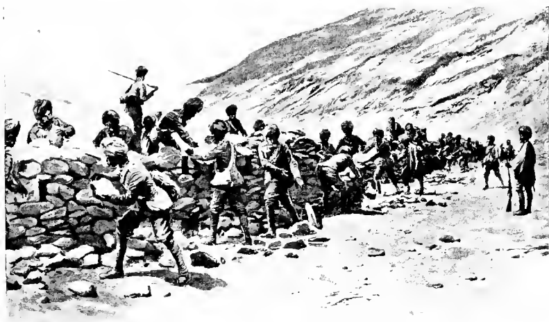
DISMANTLING LOOP-HOLED WALL AT KANGMAR
